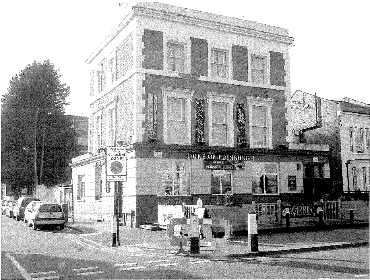
Front of premises facing Mayes road, corner of Coburg Road N22
